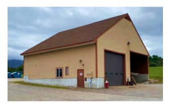
building does not have any back-up power (e.g. generator or connections for a mobile generator). This is a major concern as power from this building is used at the Town fuel pump.
