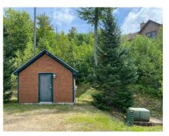
This pump station was built during the Cascade Ridge Subdivision development in 2005. The station contains two pumps used to boost water pressure to several properties located on Bean Bender Road.
