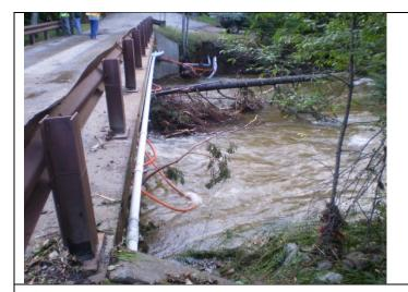
West Branch Road Bridge, Debris and utility damage on bridge.
