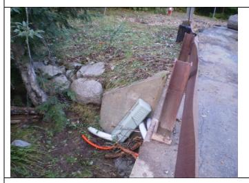
West Branch Road Bridge, Debris and utility damage on and around bridge.
